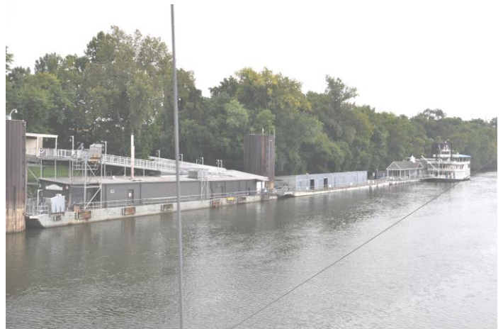
The Showboat Pier and Ramp
